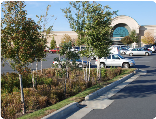
An example of a bio-retention area in a mall parking lot in Charlotte, NC. The curb cuts allow stormwater to enter the retention area.
