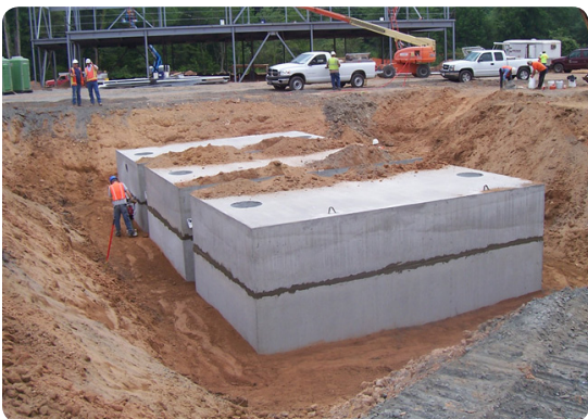
Cistern to store 60,000 gallons of rainwater for irrigation and toilet flushing at a new school on the Qualla Boundary.
