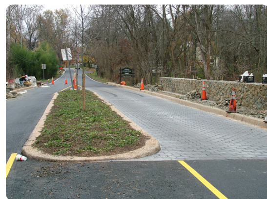
Stonework on the bridge, a traffic-calming splitter island, and textured pavement on the bridge deck provide elements of context-sensitive solutions for a rural highway in a historic corridor in Virginia. Similar design concepts could be applied in the NC 28 corridor in the Cowee Valley or other regional locations, as appropriate.
