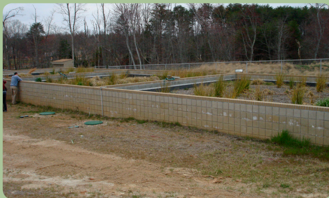
The constructed tidal wetland that is part of the Living Machine installation at North Guilford Middle School. This aerobic system functions on alternating fill and drain cycles.
