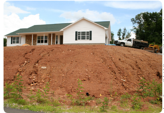
An example of a home site under construction without erosion or sediment control.
